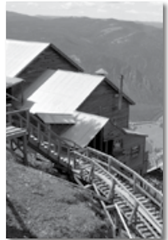
Decommissioned mine in British Columbia.
