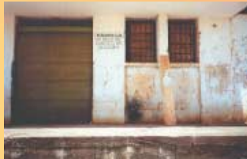
FIGURE 2: The large tracts of mono-culture plantations across Minas Gerais have played a significant role in displacing local people and jobs. This out-of-business small oil factory in Curvelos, Minas Gerais illustrates the nature of these socio-economic impacts.
