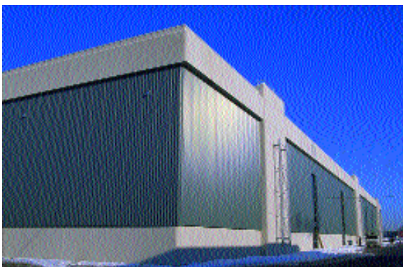
A solar thermal wall provides space heating for one of Bombardier's Montreal facilities (photo courtesy of Natural Resources Canada).
