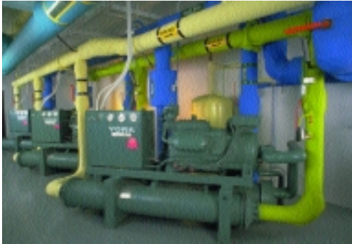
A ground-source heat pump provides earth energy to heat a building in Ottawa (Photo: courtesy Natural Resources Canada)
