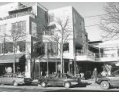
Mixed use development, geothermally heated building, Vancouver. Hotson Bakker Architects Developer: Saltlick Projects Ltd.
