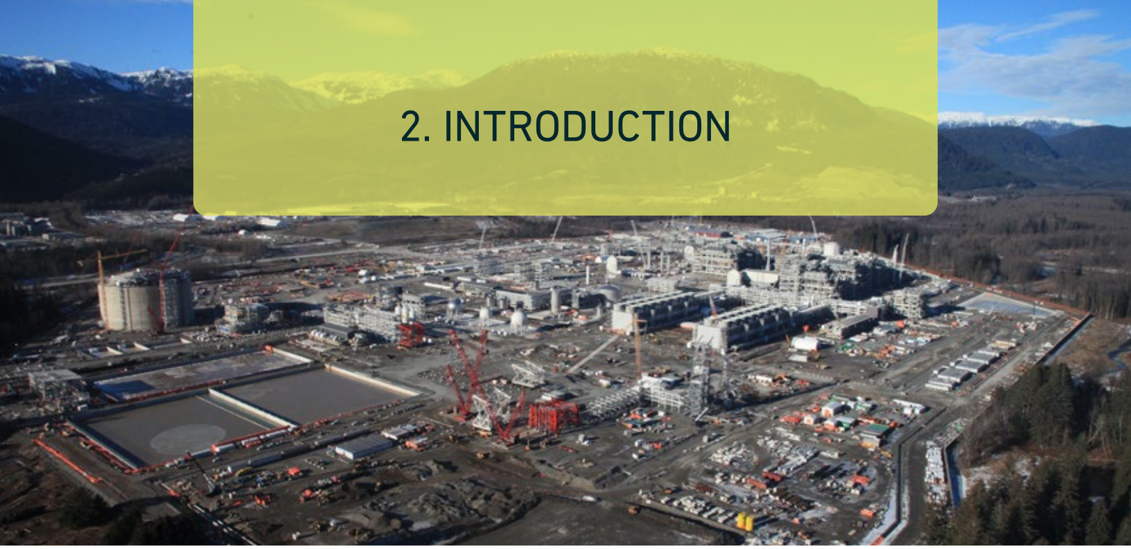
Coastal GasLink, LNG Canada. Photo: Citizen Monitoring Group
