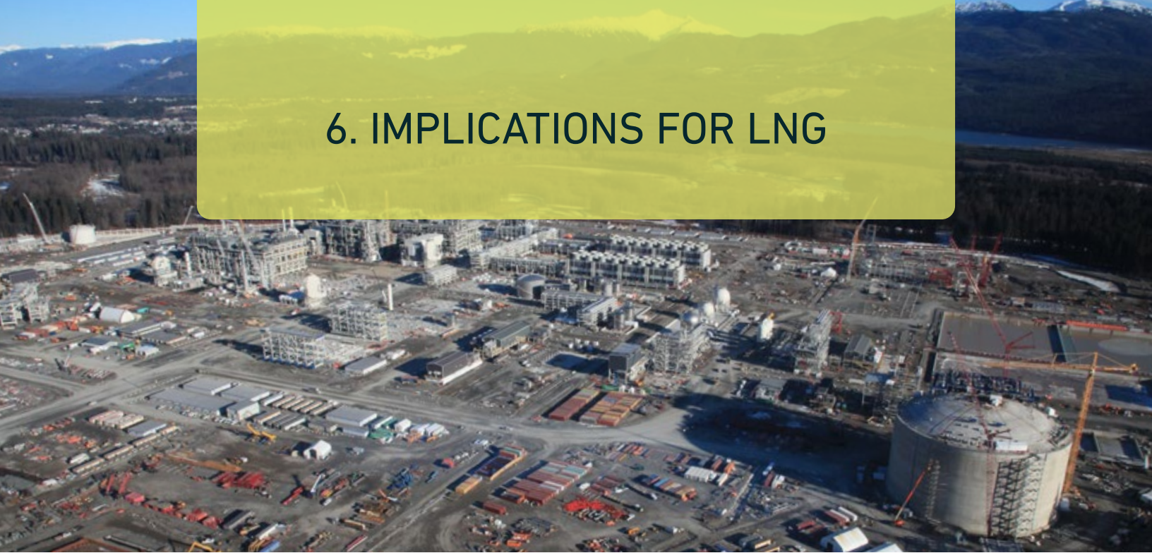
LNG Canada Construction. Photo: Citizen Monitoring Group
